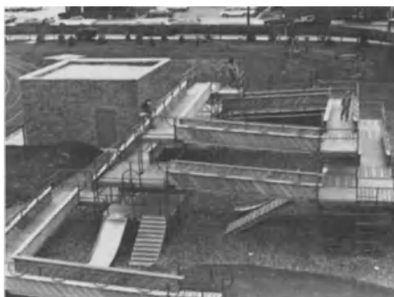
The Heights Playstructure. The continuous ramp spirals up 11 feet, forming a hollow "hill," limiting falls to short distances on the outside, and creating a "meeting place" on the inside.
